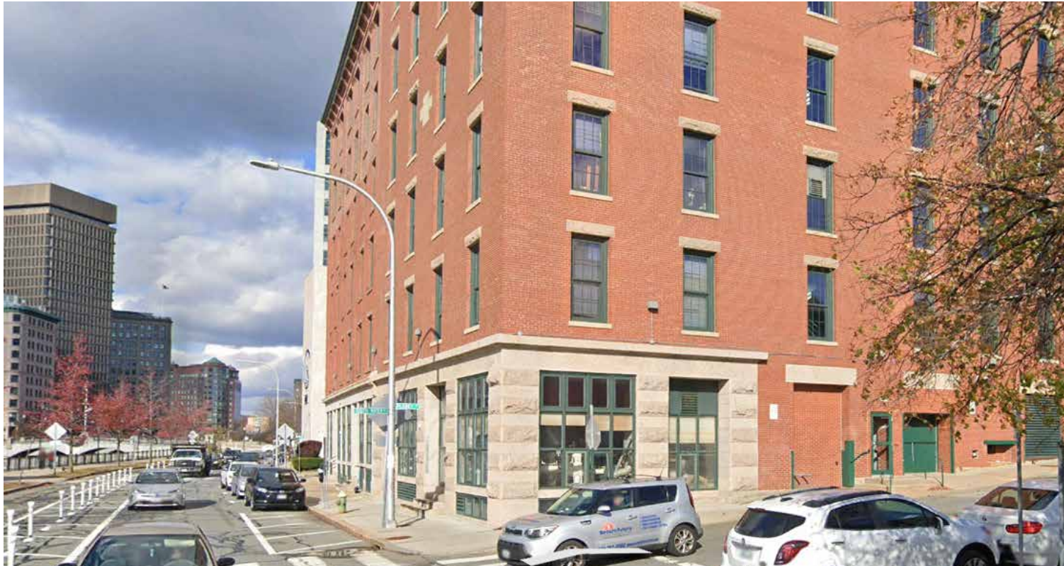
-vertically oriented punched windows in masonry wall, stone water table
