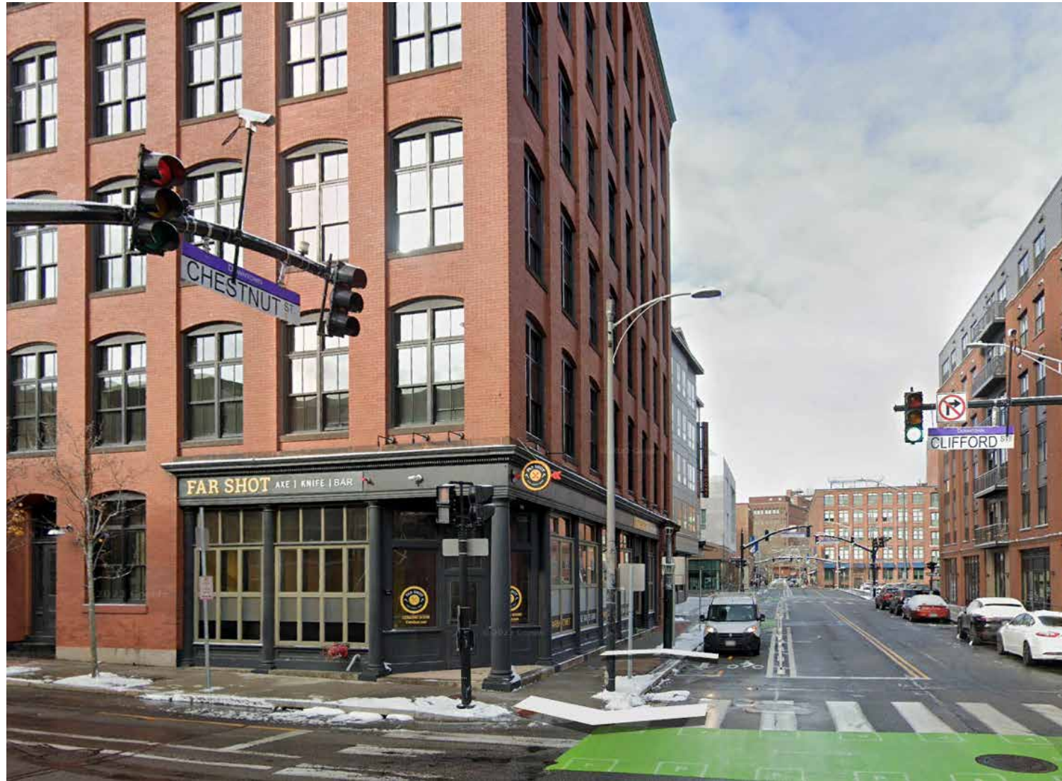
-brick pier expression extending to ground, retail base
