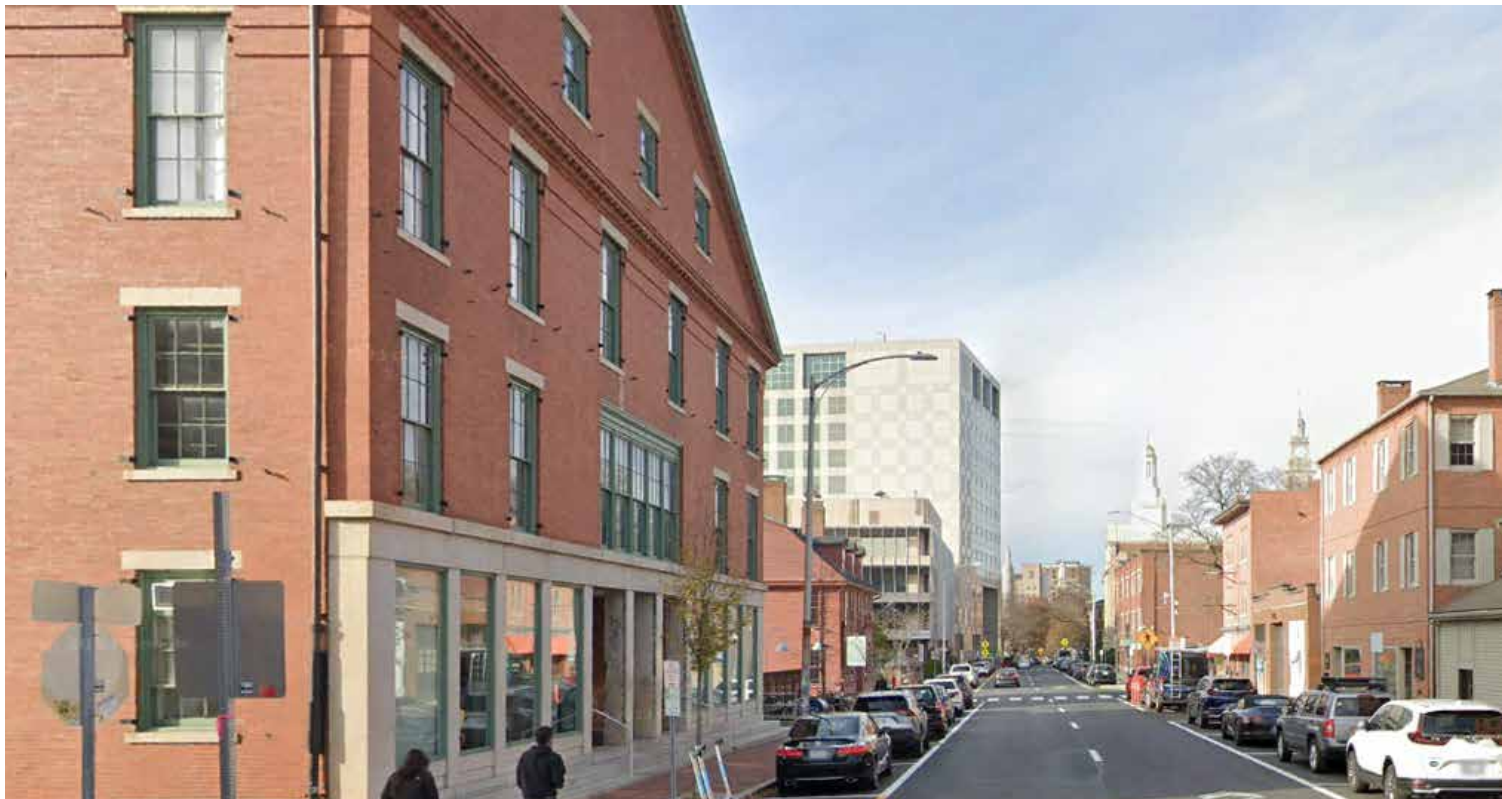
-masonry wall, lower stone retail base
